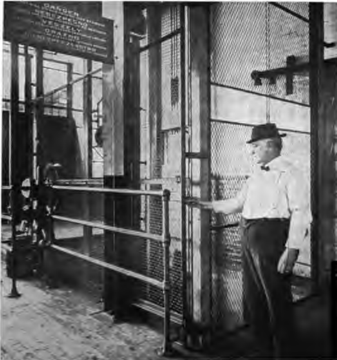
Fig. 1. Elevator Installation with Sign, Signal Button, 6' Gate, Railing around Operating Mechanism, and Enclosure of Woven Wire Fabric. The latter offers practically no obstruction to the light.*
